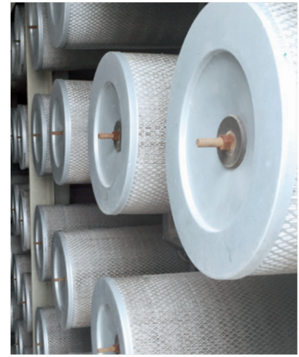
Installed GTS cartridge sets
