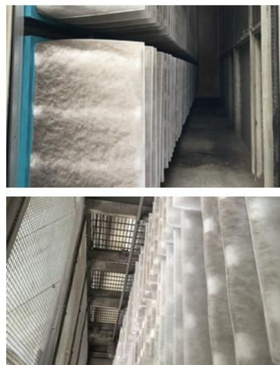
Installed hydroMaxx coalescer prefilters – the white areas on the filters (picture above) show a kind of self-cleaning effect
