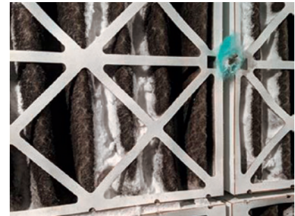
The initially installed cardboard prefilters collected snow inside the pleats resulting in clogging
