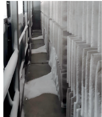
The Viledon® solution: snow slips off the filter pockets, gathering and melting on the floor
