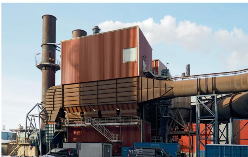
Bag filter house of Finnish steel manufacturer equipped with NEXX bags
