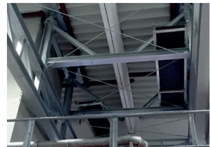
Special substructure to optimize structural rigidity of the building hall
